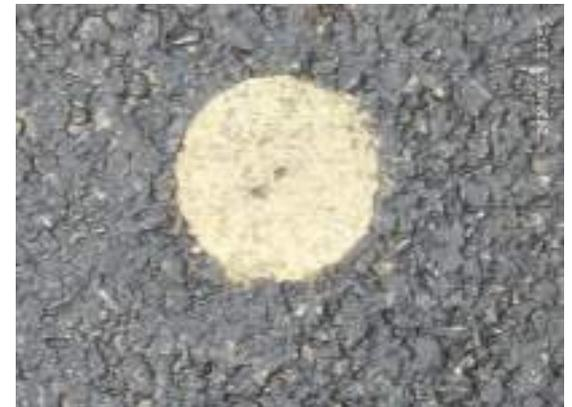
**Concreting in hole of core cutting**
