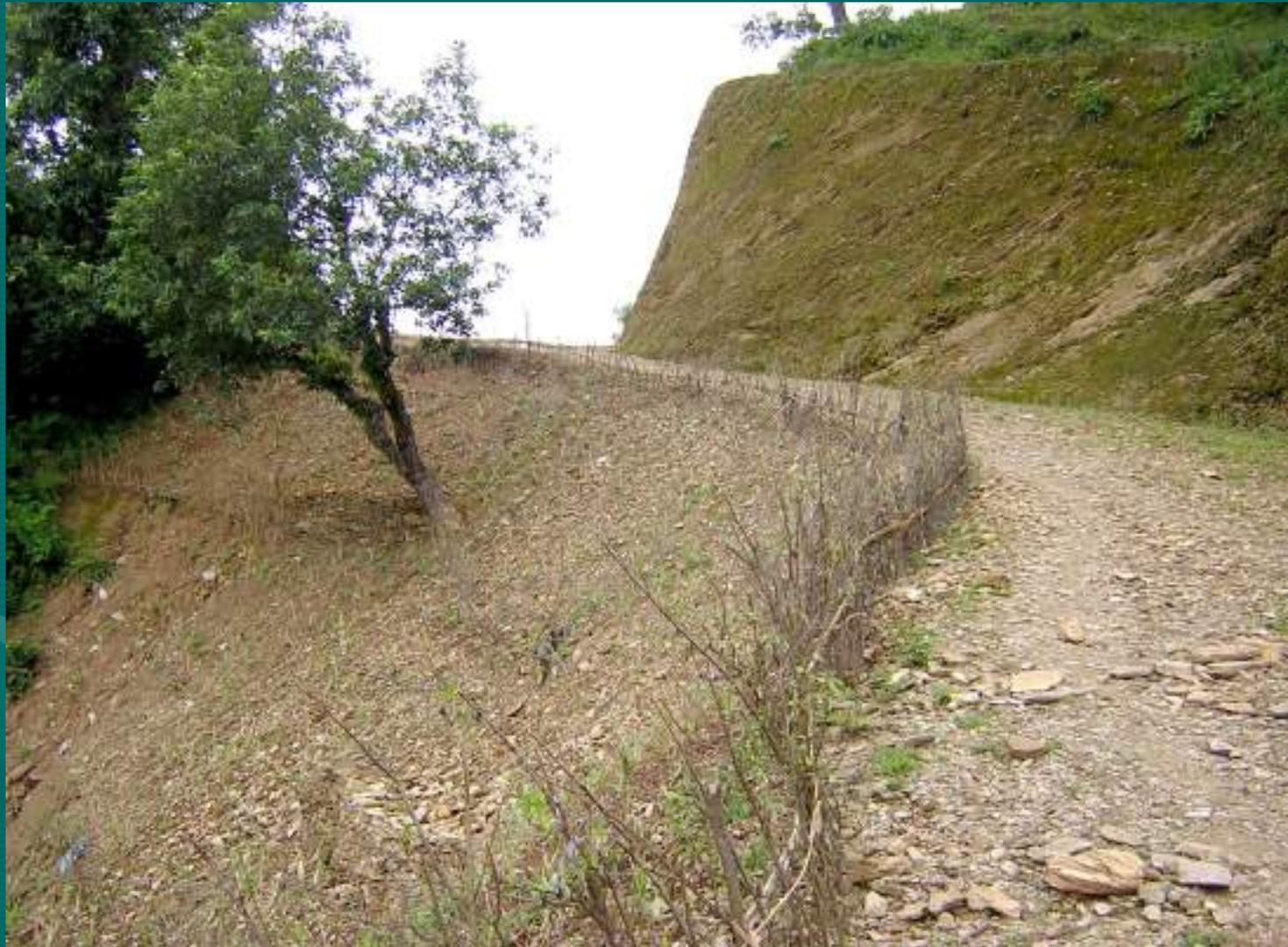
**Bio engineering work along down hill side of road section to prevent probable erosion on slope.**
